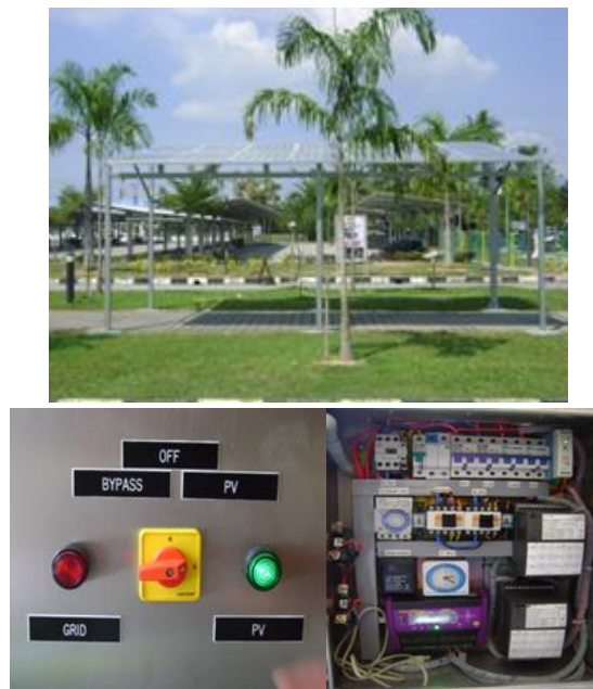
Figure 2. Dual-power PV-grid Energy System Currently Installed in UiTM Pulau Pinang, Malaysia
